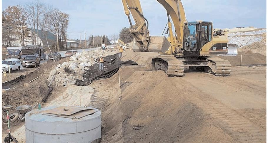
Mirafi® 180N was placed on the slope face and covered with riprap to protect the slope from erosion.
