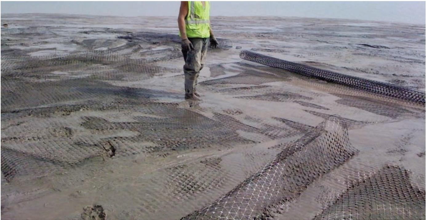
Soft soils migrate through the geogrid apertures due to its lack of separation capacity.
