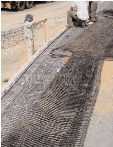
Geogrid connected to the block being staged prior to placement of backfill material.
