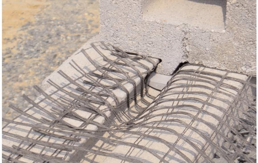
Close-up of the block/grid connection shows the lock bar in the groove providing the connection required for HITEC and VDOT.
