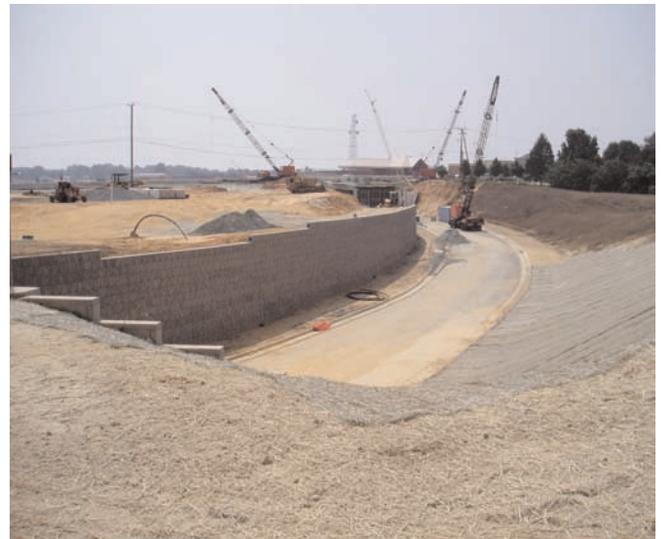
Construction of the long curved wall required between the new bridges.
