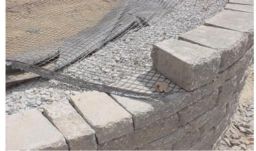
Lower retaining wall construction: Miragrid® 2XT and nonwoven filtration and drainage geotextile.
