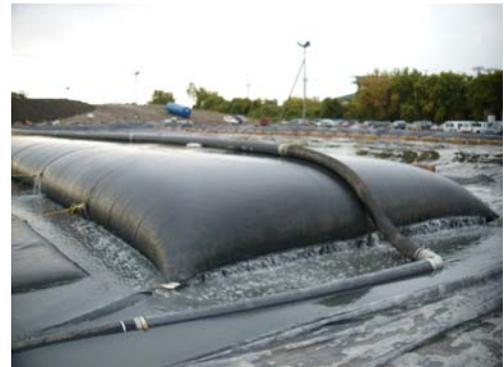
***The Conner Creek project is using 75 Geotube containers to collect contaminated sediments.***
