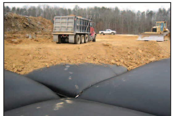
When moisture content reached 35 percent, the tubes were covered for reclamation.
