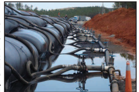
A manifold system was used to control the flow between the Geotube® units.
