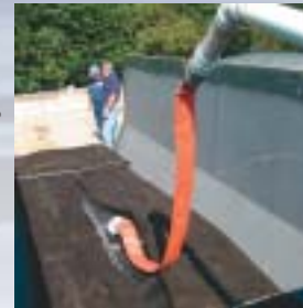
Sludge is pumped into the Geotube® MDS™ unit for dewatering.
