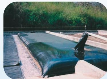
Under proper conditions, Geotube® MT units can also be used in drying beds to increase capacity.
