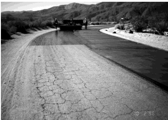
24 Photograph 2. Fabric Placement on Roadway with Sound Structural Section
