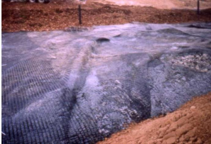
Figure 4. Geogrid Deformation
