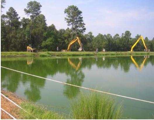
Figure 8. Backhoes and bobcats were used to pull the geotextile across the water.
