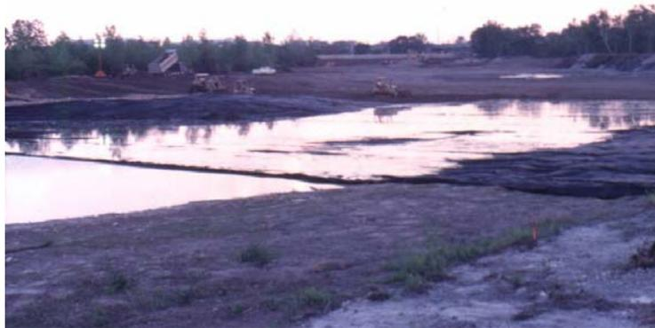
Figure 11. Monofilament Geotextile In Place for Construction Platform
