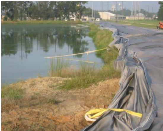
Figure 6. Geotextile was sewn together on land and accordion folded. Pulling points were established 35 meters apart.
