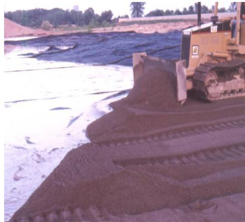
Figure 14. Initial Fill Placement Lift is 1/2 m
