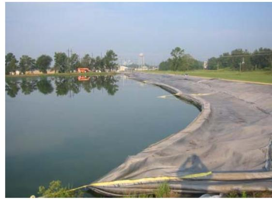
Figure 9. The manufactured specific gravity of the geotextile of 1.07 allowed it to float long enough.
