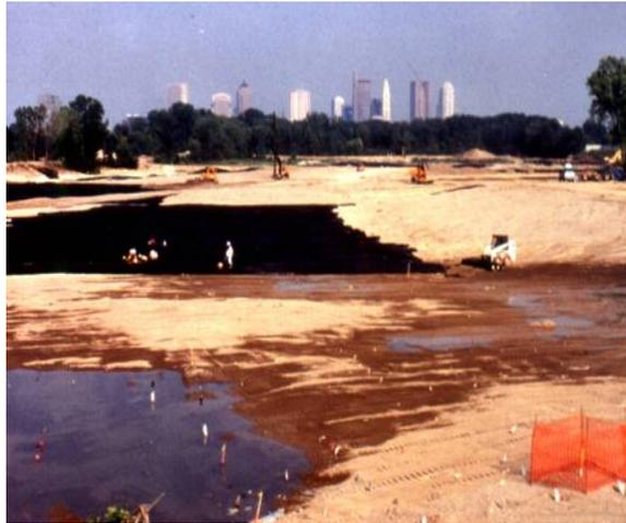
Figure 12. Initial High Strength Geotextile Layer, With Wick Drains Shown In Foreground
