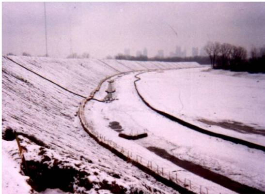
Figure 15. 12 m High Embankment with 2H:1V Side Slopes In Place
