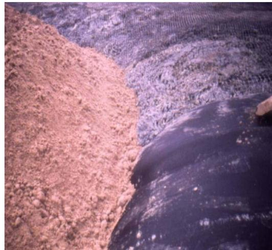
Figure 3. Fill Placement with Mud Wave
