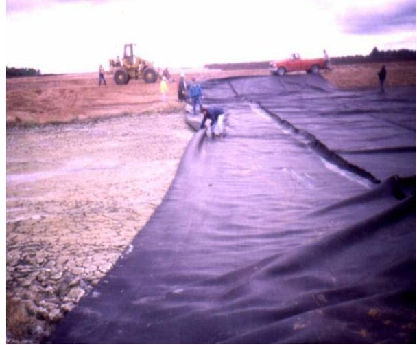
Figure 2. Geogrid and Geotextile Deployment
