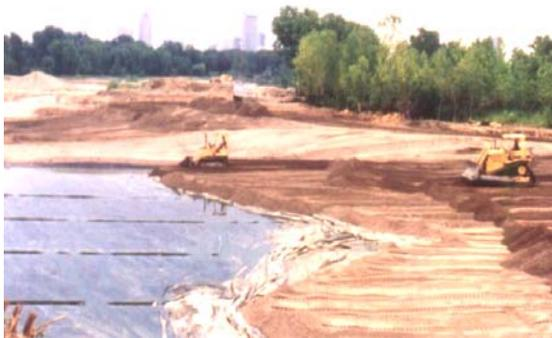
Figure 13. Smaller Dozer On Leading Front Attempts to Limit Mud Wave Formation
