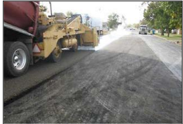
Figure 3. Sanded fabric (right) and construction of second chip seal.
